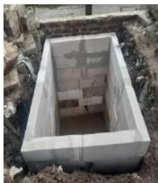
Rehabilitasi MCK Pasar Semampir
