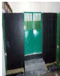
Rehabilitasi Mushola Pasar Bantul Lantai 2
