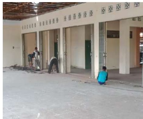
Rehabilitasi Pasar Bantul
