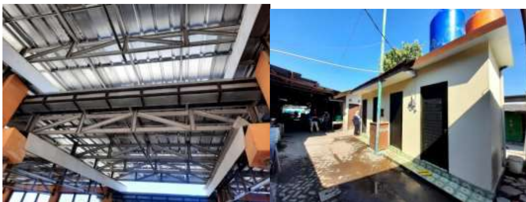
Rehabilitasi Pasar Bantul
